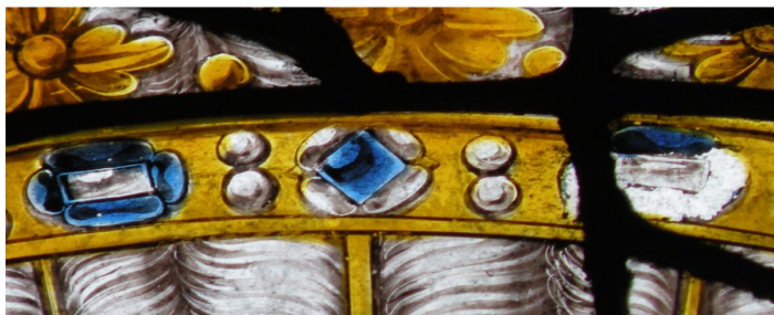
Failing blue enamel Hamsterley Hall
